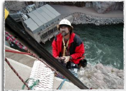
Reed Thorne working on rope with Jayne Thorne on Salt River Project Horse Mesa dam inspection 1999
