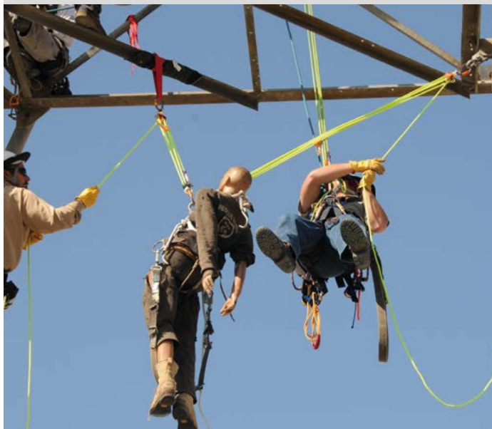
BELOW: Linemen using several jiggers to transfer a mannequin across the bottom of a transmission tower.
