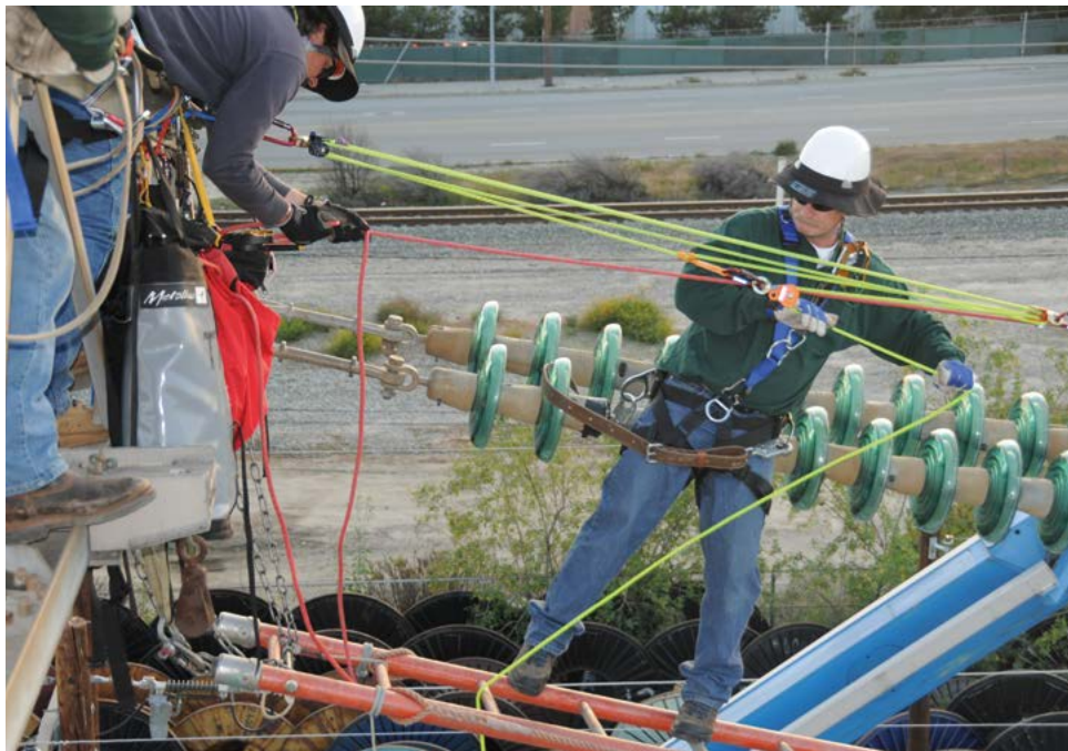
ABOVE-LEFT: A Los Angeles Dept of Water & Power lineman standing on an aerial ladder uses an AZTEK high on a power line to lift 2 men off the conductor using both prusiks (blue as the ratchet and orange as the haul grab) for an 11:1 complex mechanical advantage. Similarly, a 12:1 compound pulley system (noted 3:1 x 4:1) can be had by simply turning this one around end to end.
