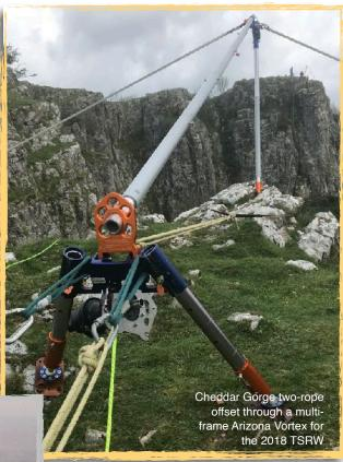
alternatives to highlines in the form of 'offsets'. In the past 20 years, RTR was instrumental for championing high angle offsets as an alternative to training-intensive highlines. Offsets employ standard high angle techniques that most rescuers already know and so are more forgiving in the training curve than highlines.
